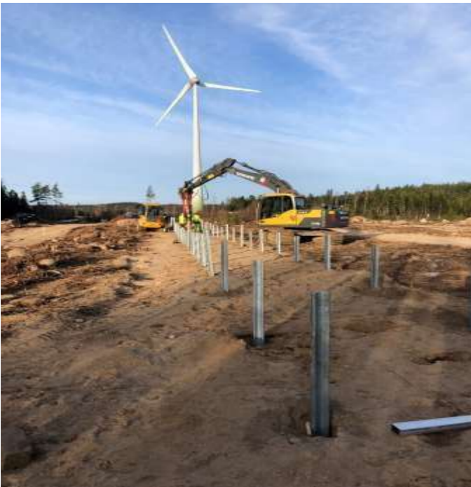
Markstativen monteras
