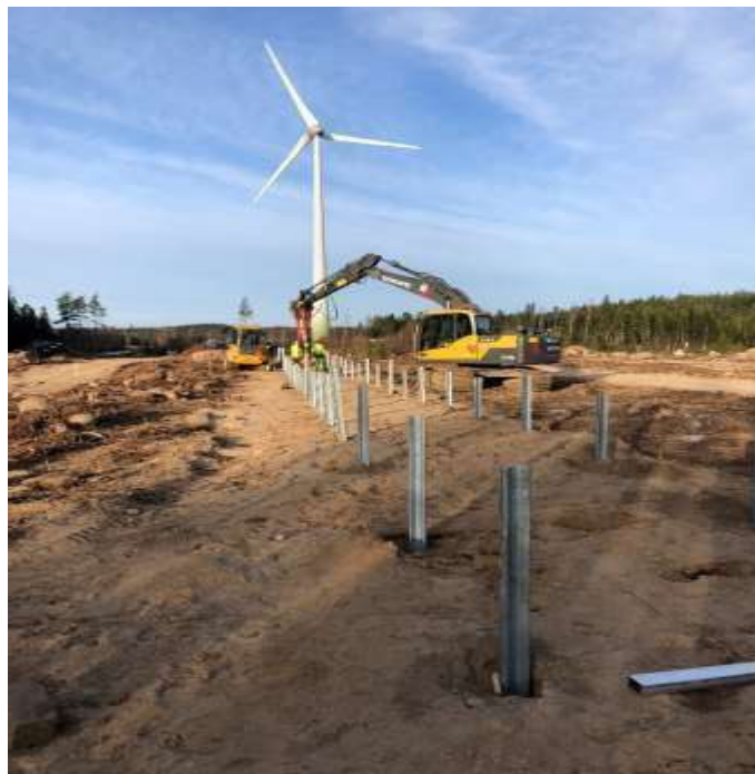
Markstativen monteras
